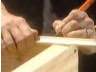
Hold the cove moulding in place and mark the length
