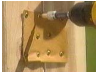
Attach the hinge with 'pan head' screws
