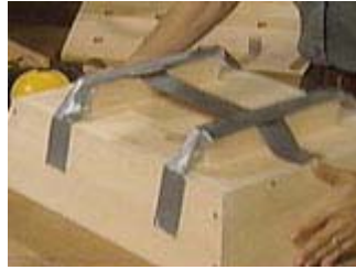
Glue 'em, then tape them in place until dry
