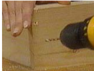
Pre-drill before nailing
