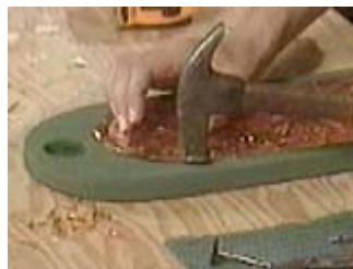
Tack it in place with half inch copper nails
