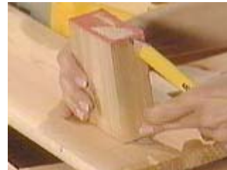
Put a scrap piece of 2x4 in the marked corner and trace the shape for cutting
