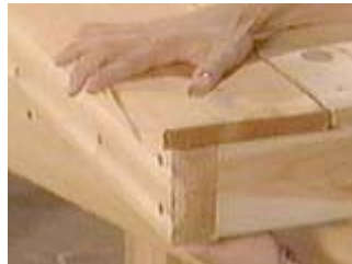
Put the board in place and mark the corner from underneath
