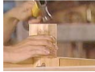
Use a hammer and block of wood to tap it into place if necessary
