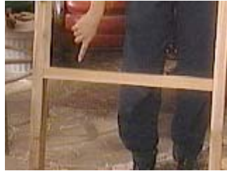
Add a 2x4 deck support in the center of the frame
