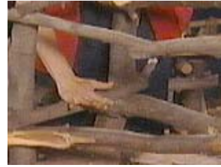
Attach the front to the back with some cross pieces
