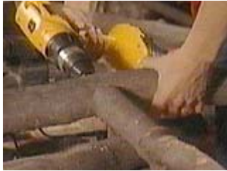
Pre-drill for the nails
