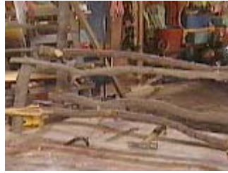
The completed front frame standing with the back
