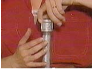
Attach a three quarter inch galvanized coupling to the short pipe.
