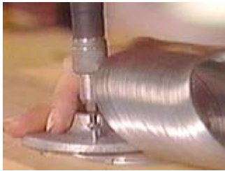
Attach the flange with screws over the end of the slinky.
