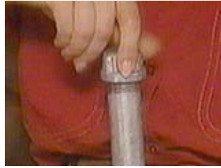
Put a cap on the end of the short pipe to protect the threads.
