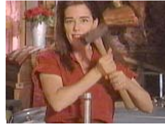
Drive the capped short pipe into the ground using a sledge hammer.
