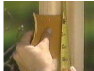
Set hinges about 11 inches from the ends, plus one in the middle
