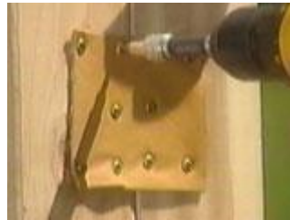
Attach the hinge with 'pan head' screws
