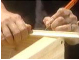
Hold the cove moulding in place and mark the length
