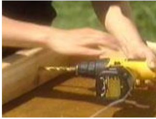
Start the drill straight to drill an angled hole
