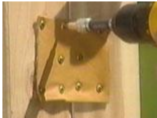
Attach the hinge with 'pan head' screws
