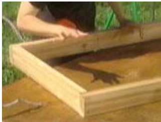
Screw the corners of the frame together
