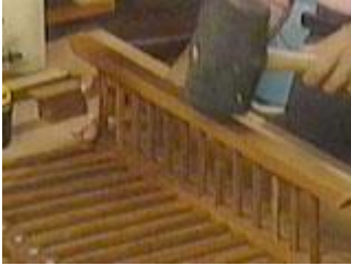
Use a rubber mallet to help seat the dowels
