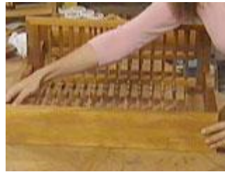
Glue and nail all the pieces in place
