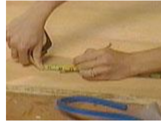
Mark the height for the seat
