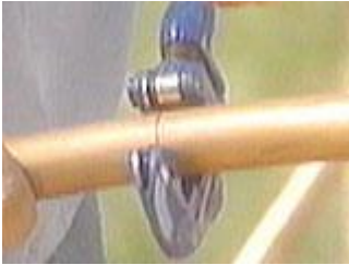
Cut it to fit with a pipe cutter
