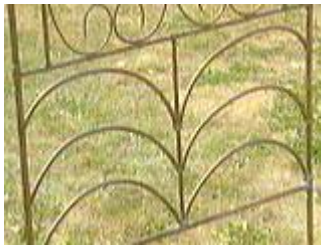
Detail - bottom of large trellis
