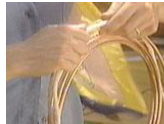
Transfer the length to the tubing
