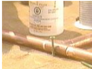
Use screws to help hold the pieces in position for soldering
