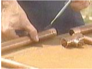
Brush the solder on the outside of the tubing
