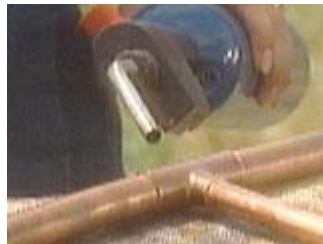
Use a plumber's torch to heat the joint
