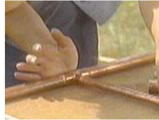
Push the pieces firmly together
