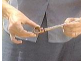
Brush the flux on the inside of the fittings
