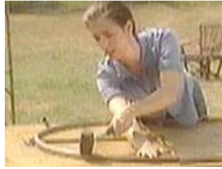
Use a rubber mallet to take the waves out
