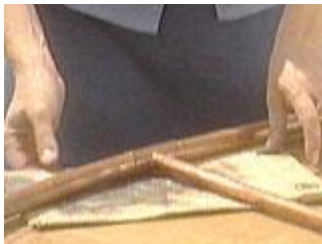
Place a plumber's fire proof mat under the joint to be soldered
