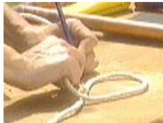
Mark the length on the sash cord
