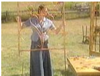
Slide the trellis over half inch re-bar set in ground
