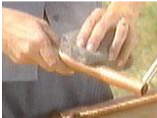
Steel wool will quickly clean the tubing, removing manufacturer's info
