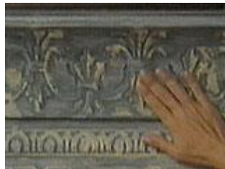
Detail of crown molding and trim
