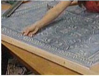
Place the trim and tack the pieces in place with escutcheon pins
