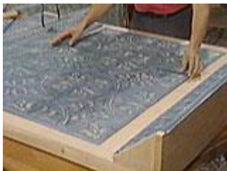
Place the centre panels leaving room for the trim
