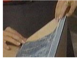
Attach it in place with glue, screws and nails
