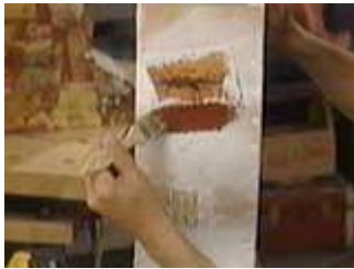
Paint the plaster with milk paint
