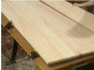
Place the four boards in pipe clamps
