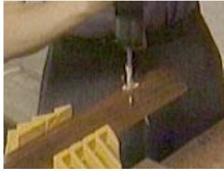
Pre-drill for the hanger bolts
