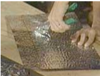
Then use tinsnips to cut out the centre section
