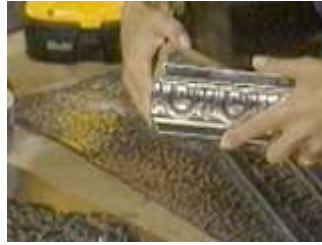
Cut the outside corners to fit snugly
