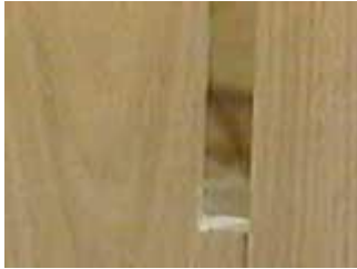
If the legs wobble on a flat surface, file one of the slots a bit
