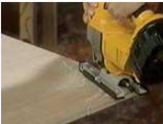
Cut along the lines with a jigsaw
