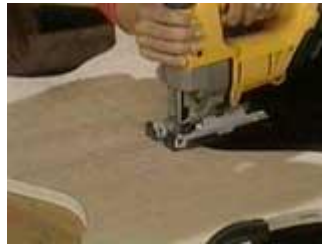
Mark and cut out the second slot
