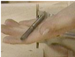
Use the hanger bolt to mark the location to drill
