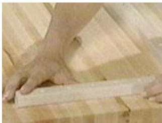
Put the blocks in place and attach with screws
