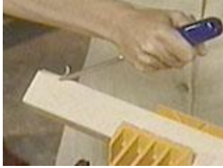
Make a flat spot on the inside corner of the legs
