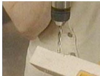
Drill for the hanger bolt
