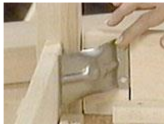
Cut the slots for the leg braces
