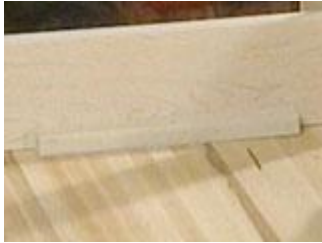
Make one-inch strips to support the apron
