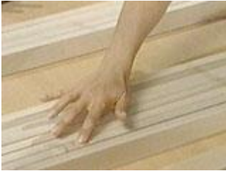
Sort the boards putting knots down
