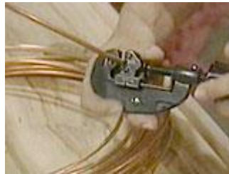
Cut the copper with a tube cutter
