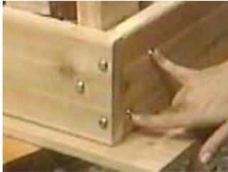
Put the 2x4 legs in place and attach with staggered screws
