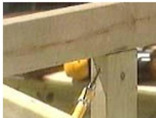
Toe-screw a center support to the back
