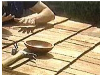
Determine the shingle exposure by measuring and dividing the roof top distance
