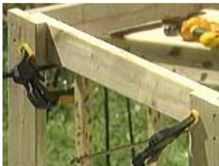
Attach using three inch zinc screws
