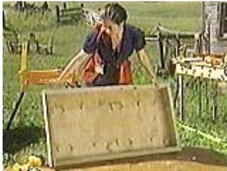
Make a floor out of pressure treated 2x4 and exterior grade half inch plywood
