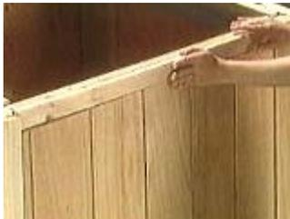
Cut the doors to fit inside the trim and one half to one inch off the ground
