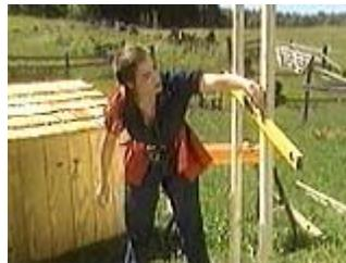
Mark the pitch angle on the posts and cut on the line
