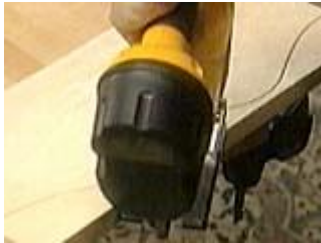
Use a jig saw to cut out the pieces
