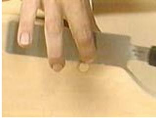
Cut off the plugs with a flush cut saw
