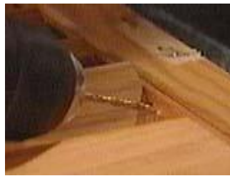
Pre-drill for the screws
