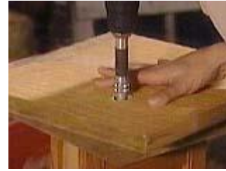
Attach the lazy Susan to the smaller base through the peephole
