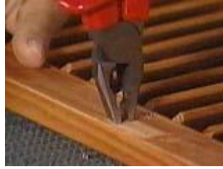
Use pliers to back out the headless screw
