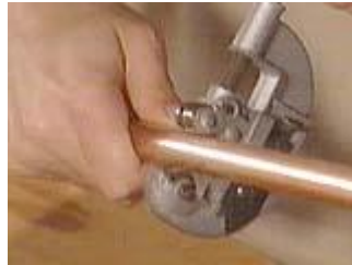
Use the pipe cutter to cut the lengths of pipe
