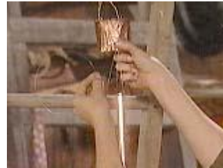
Hang the copper circle and tie the pipes to it
