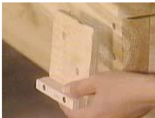
Make a smaller jig to locate the holes for the carriage bolts on the lower deck
