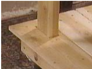
Cut a hole in the deck to accept the leg
