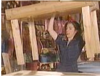
Set the top section in place over the bottom section
