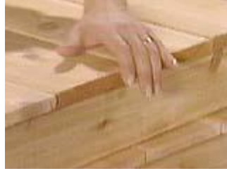
Even them up using your fingers to measure an equal overhang on each side
