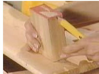
Put a scrap piece of 2x4 in the marked corner and trace the shape for cutting
