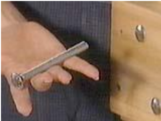
Attach the legs with carriage bolts
