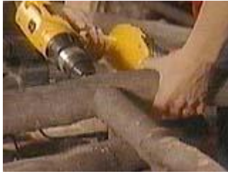
Pre-drill for the nails
