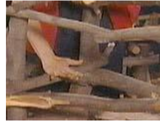
Attach the front to the back with some cross pieces
