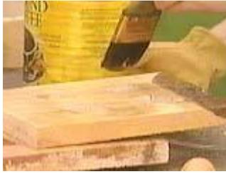
Brush on the stain before attaching the sides together
