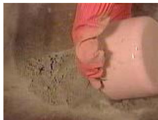
Measure one part cement into the bottom of the wheelbarrow
