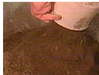
Putting the other ingredients over the cement keeps the dust down
