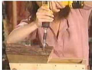
Attach the top front piece with screws
