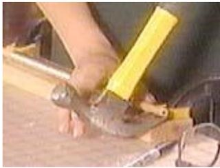
After drilling, use a hammer to pry the tube and doweling up
