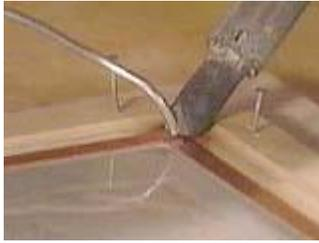
Heat the joint and add the solder when hot
