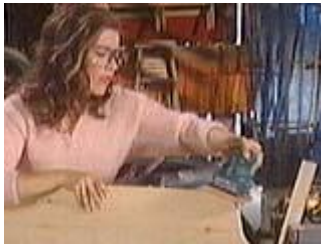
Sand out the rough spots
