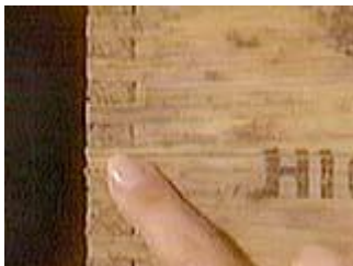
Box joints on an antique box
