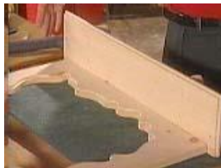
Center the shelf under the mirror and attach it with screws
