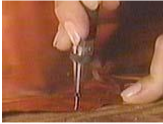
Use a compression punch to make dimples in the metal for drilling
