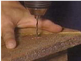
Pre drill before driving the nails in
