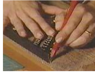
Use a speed square and pencil to mark the 45-degree cut line
