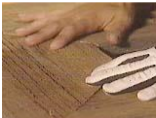
Fit the pieces together before gluing
