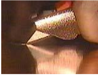
At the mark cut two slits in the reflector the width of the tab
