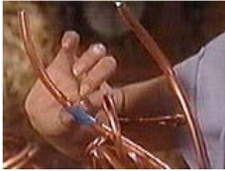
Mark the pipe that will carry the electrical wire so as not to drill into it
