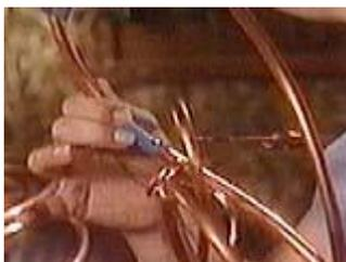
Use emery paper to remove oxidation prior to soldering
