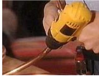
Drill holes in the larger pipe to help attach the smaller ones
