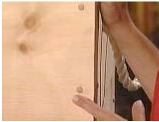
Use wooden plugs to cover the screw heads.
