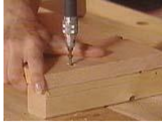
Attach the sides, front and back to the corner post with screws.
