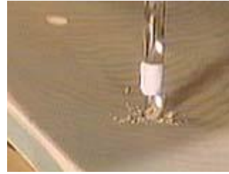
Drill the holes on the marks
