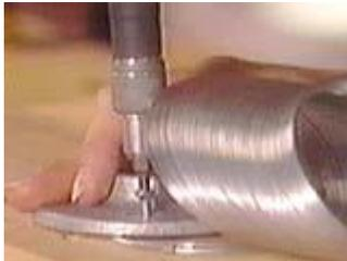
Attach the flange with screws over the end of the slinky.
