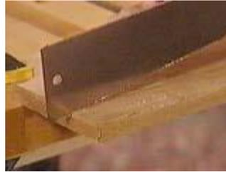
'Rip' a board to one and one half inches using a rip saw.
