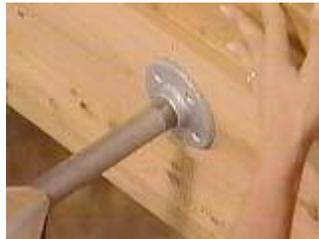
Galvanized flange and pipe attached to the tray.
