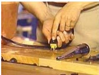
Now slide the housing over the connected wires, securing it with the provided screw.
