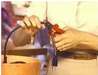
Next, cut the plug off the pump. This will give you a severe emotional spike, since you are effectively wrecking your \$50 pump. However, it is really a minor act of derring-do, since you will now re-wire the cord using your replacement plug.
